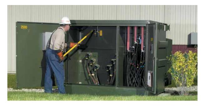
Cooper Power Systems three-phase pad-mounted transformers are available in live-front or dead front designs. Design include delta and wye configurations with single or series multiple combinations with either taps or notaps. In an underground primary feeder system, three-phase pad-mounted transformers are an alternative to three-phase substation transformers
